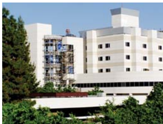
PHOTO COURTESY OF SEALS/BIEHLE GENERAL CONTRACTORS.
